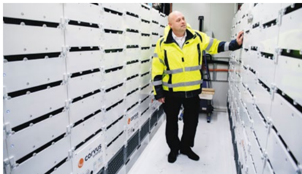
Above: Johan Stranne inside the battery unit. Right: The 1 MWh battery unit, equal to the power of about 12 Tesla cars and with a weight of 30 tonnes, is placed on the weather deck to fit.
